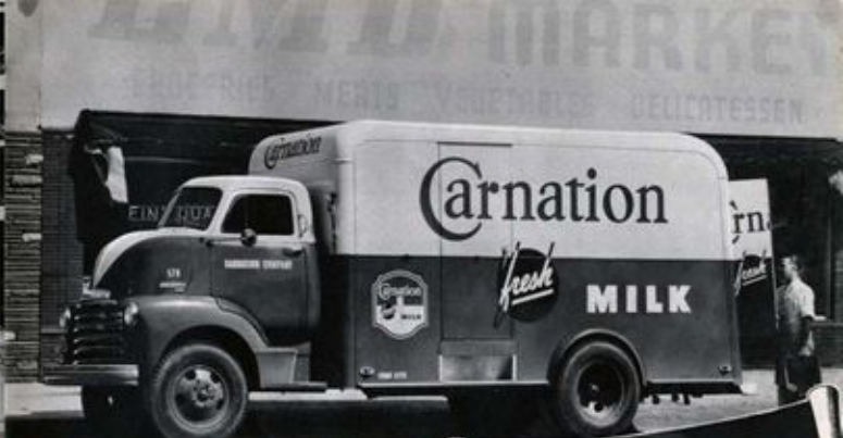
MODEL 3703 Chassis and Cab 118" WHEELBASE, MAX. G.V.W. 16,000 LBS
