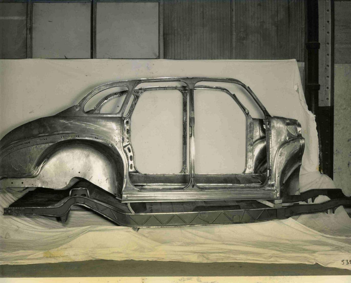
Unit body construction principles will be employed by Nash for all its 1941 models. This gives you an idea of how they are built. Sides, floor, roof, back and front bulkhead are welded together into a single unit which is stronger, safer and lighter. Boxed, bridge-like girders are used, and the best of light-weight steels are employed. These bodies are built something like the light-weight streamlined trains, it is said. This picture shows the sides and floor before being welded.
