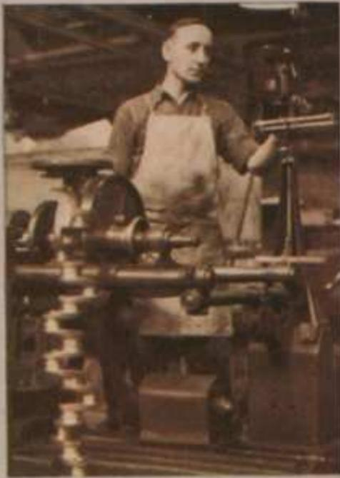
Nash-built cars represent the finest in precision engineering. Here, a skilled expert is balancing a crankshaft—one of the hundreds of tests that insures a "sweet-running" motor, free from vibration.
