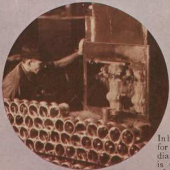
In boring pistons for Nash cars, a diamond cutter is used instead of an ordinary steel cutter. Accuracy cannot vary more than  $\frac{1}{4}$  of  $\frac{1}{1,000}$  of an inch from standard.
